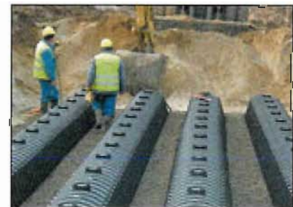
Zona industrial, Raben (PL)
