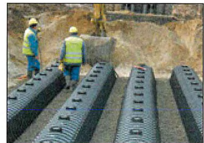
Zona industrial, Raben (PL)
